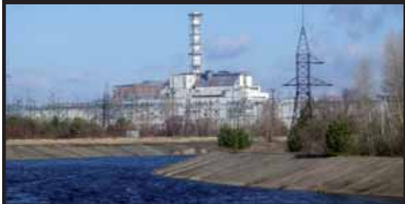
View of the damaged Chernobyl nuclear plant reactor from the Pripyat River
